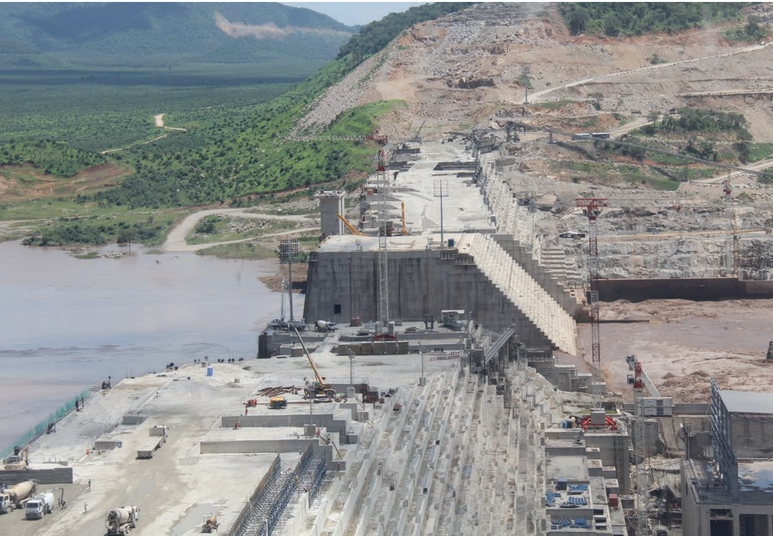
> THE MAIN DAM OF THE GERD CONSTRUCTION PROJECT ON 31 JULY, 2016.
