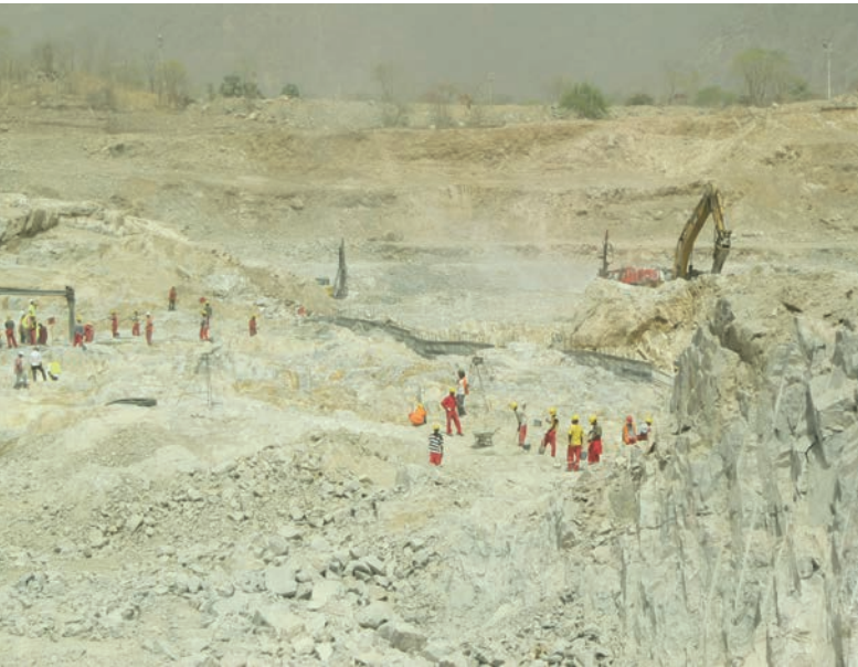
> BEGINNING OF FOUNDATION WORKS OF THE GERD MAIN DAM February 2013 © Ana Elisa Cascão
