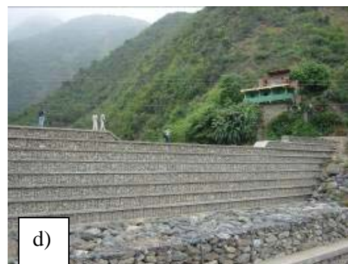
Figure 5. Different types of sediment control dams in the State of Vargas: a) a 4 m high reinforced-concrete slit dam in Quebrada Guanape; b) a 4 m high cyclopean-concrete slit dam in Quebrada Curucuti; c) a 3 m high gabion slit dam in Quebrada El Cojo; and d) a 7 m high gabion closed dam in Quebrada San Jose de Galipan.
