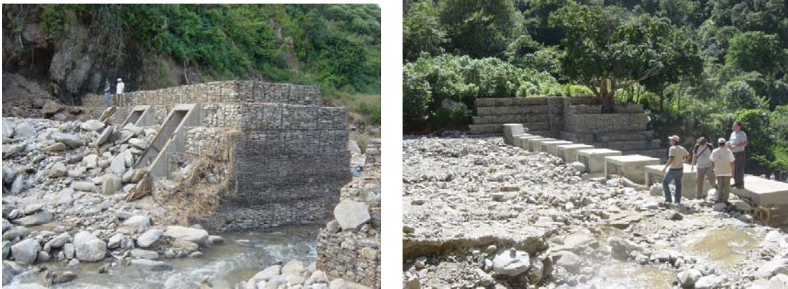
Figure 6. View from upstream of Camurí Chico window dam (left) and El Cojo dam (right).
