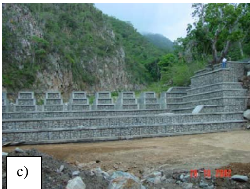
Figure 5. Different types of sediment control dams in the State of Vargas: a) a 4 m high reinforced-concrete slit dam in Quebrada Guanape; b) a 4 m high cyclopean-concrete slit dam in Quebrada Curucuti; c) a 3 m high gabion slit dam in Quebrada El Cojo; and d) a 7 m high gabion closed dam in Quebrada San Jose de Galipan.
