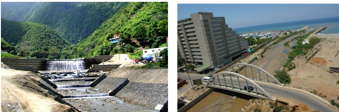
Figure 7. Canalization of San Jose de Galipan stream (left) and Tacagua stream (right) in the State of Vargas..
