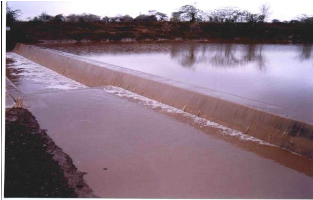
Plate – 1 Checkdam Across A River
