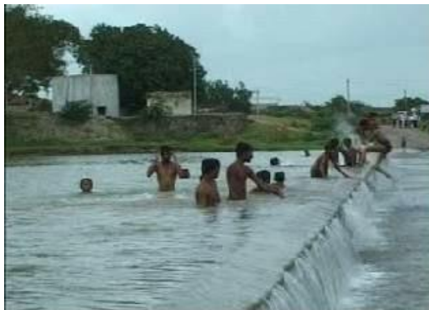
Plate – 2 Checkdam Across A River
