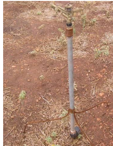
Figure 6 : Manufacturing quality of fittings and riser (2 months old sprinkler)
