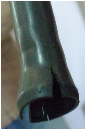
Figure 3: Pipe cracking after only 2 years' use, Syria 2002.
