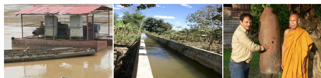
Fig 4. Floating pump and field channel for delivery of water
