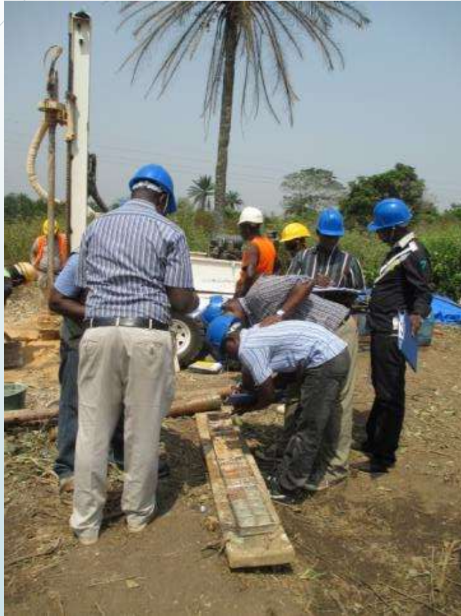
Image: Learning about sampling drilling cuttings at the drilling supervision course in Sierra Leone, 2014 (Source: Kerstin Danert).
