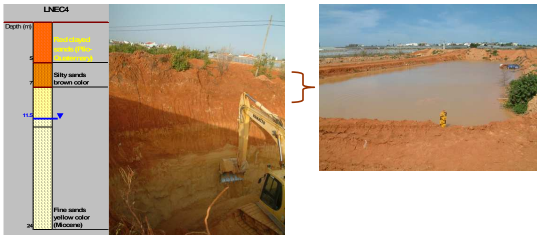
Figure 9 –Vertical profile of lithological materials in Areal Gordo (at right) and LNEC4 well lithological column and, infiltration basin in the first layer (at left)
