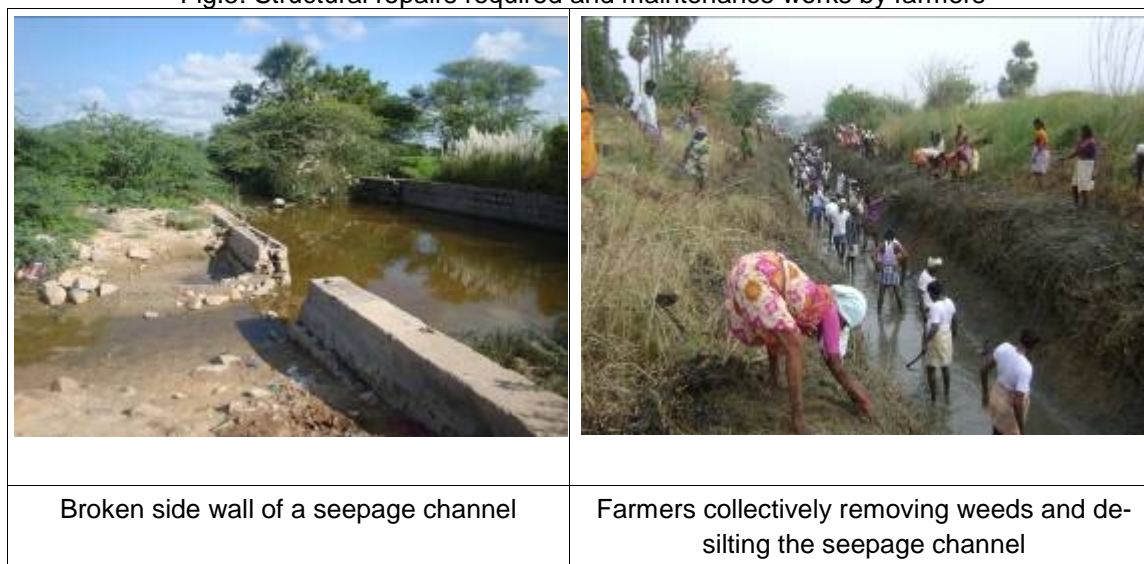
Fig.5: Structural repairs required and maintenance works by farmers
