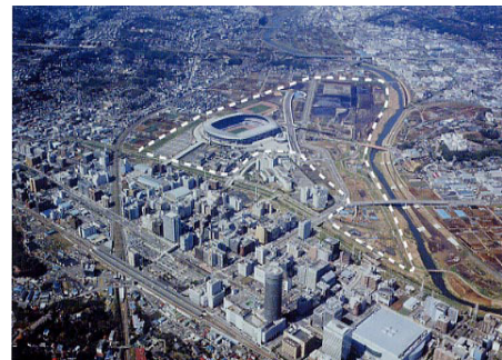
Figure. 9 Multi-purpose water retarding area for the Tsurumi River
