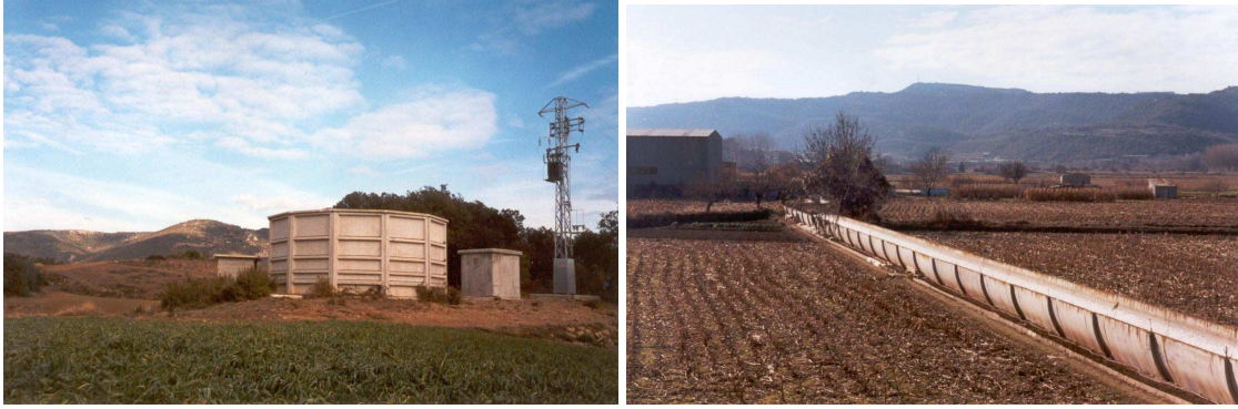
Figure 7. New water tank and irrigation ditch in Baronía and Ponts
