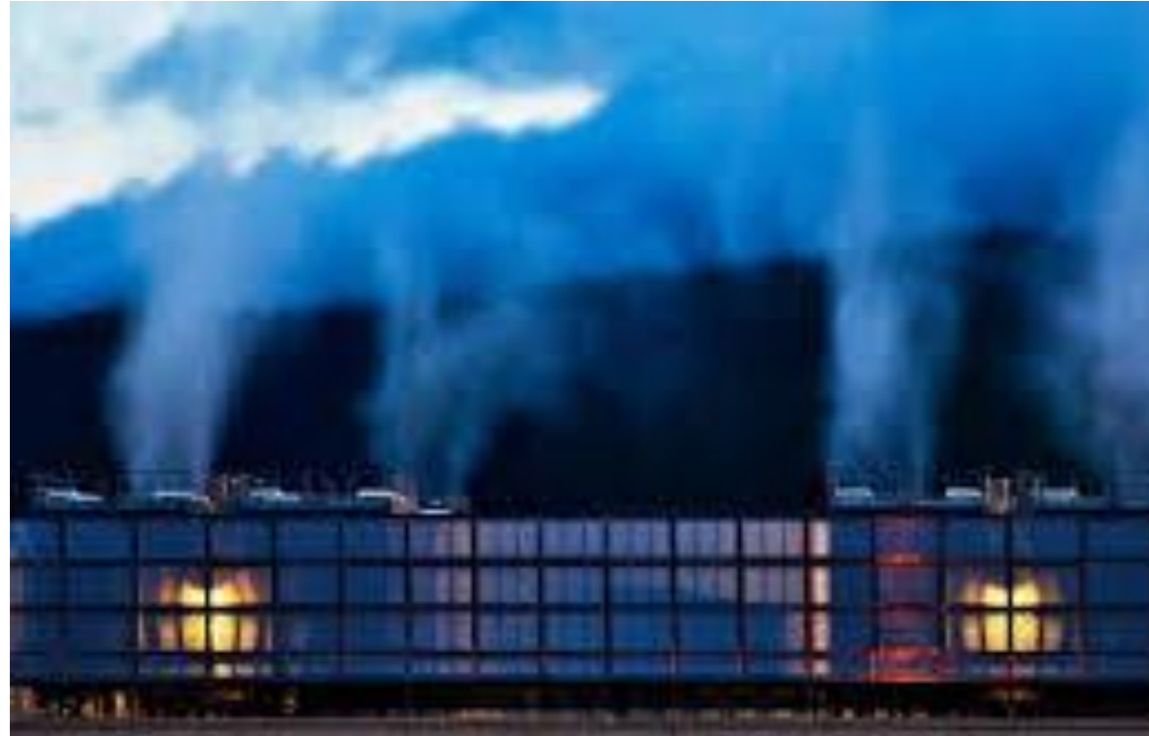
Source: Google. Data center in The Dalles, Oregon.
