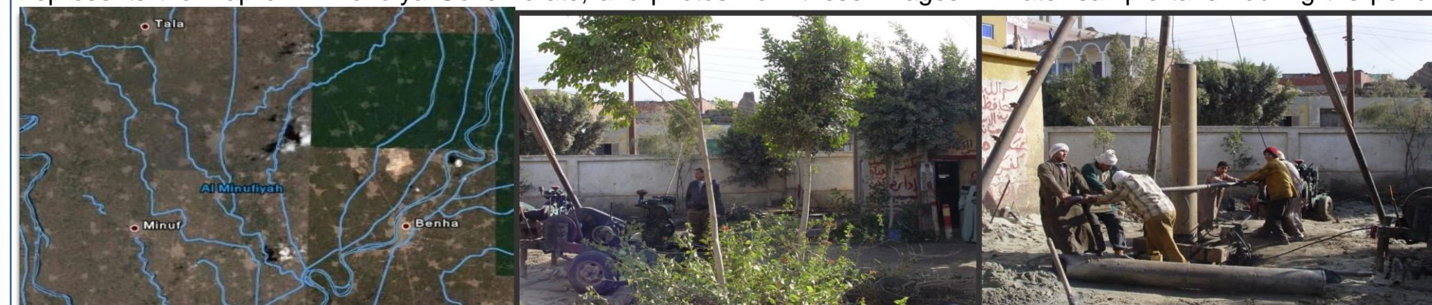
Figure 3 : Map of El Menofya Governorate – Photo Shnway Village – Drilling well at Shnway
