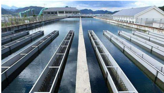
Drinking water treatment plant
