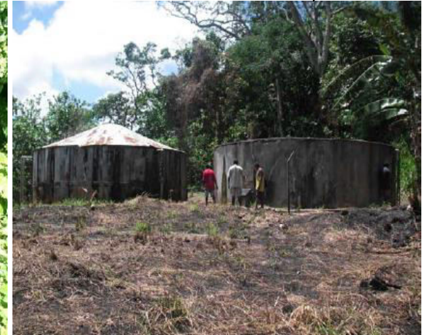
Creek water input located at Mele uphill (left) and concrete & galvanised storage tanks for Mele rural water supply. Source: Nath et al., 2006.
