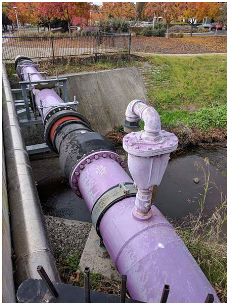
Purple-coded pipes for reuse
