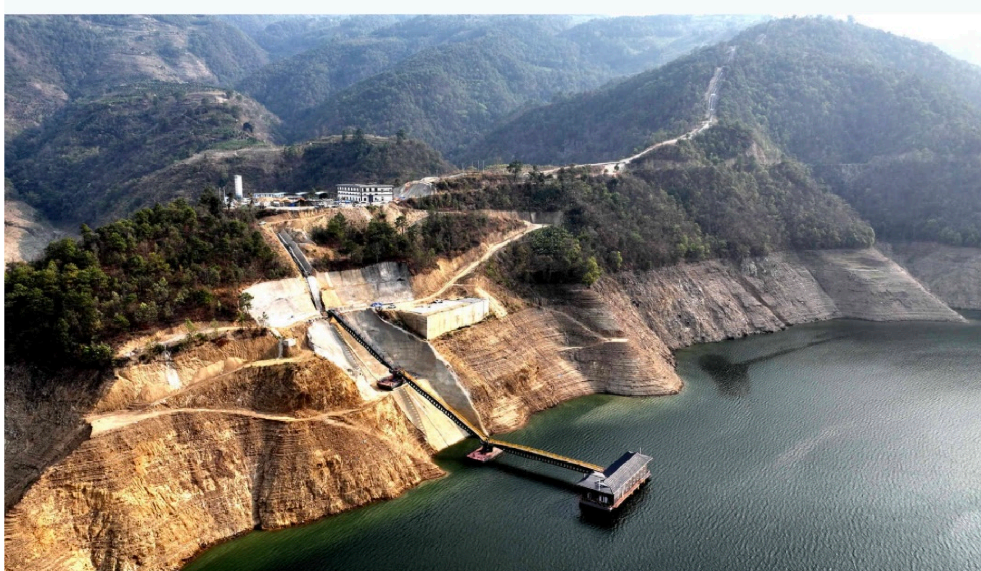
Figure 3. Aerial view of floating boat pump station
