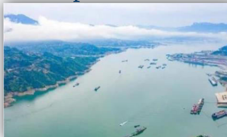
Local rainstorm and flood
