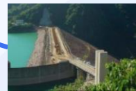
土石坝 Earth and rock-fill dam
