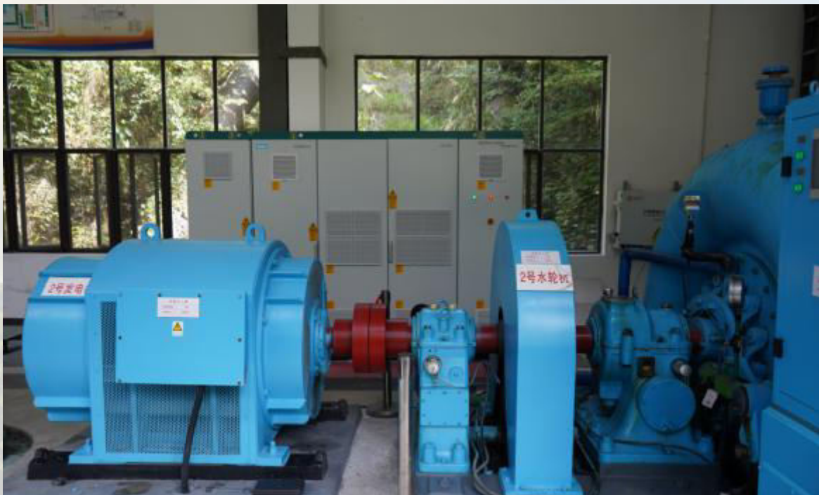
国内首台直驱型变速改造的水电机组 the first domestic direct-drive variable-speed transformation of hydropower units
