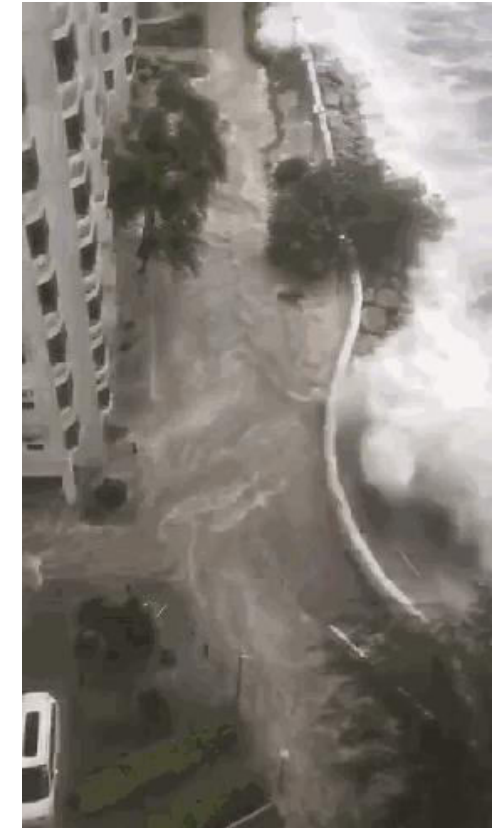
Storm surge and wave overtopping during Hato (Hong Kong)
