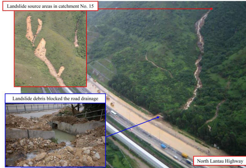
North Lantau Highway flood due to drainage blockage by landslide debris
