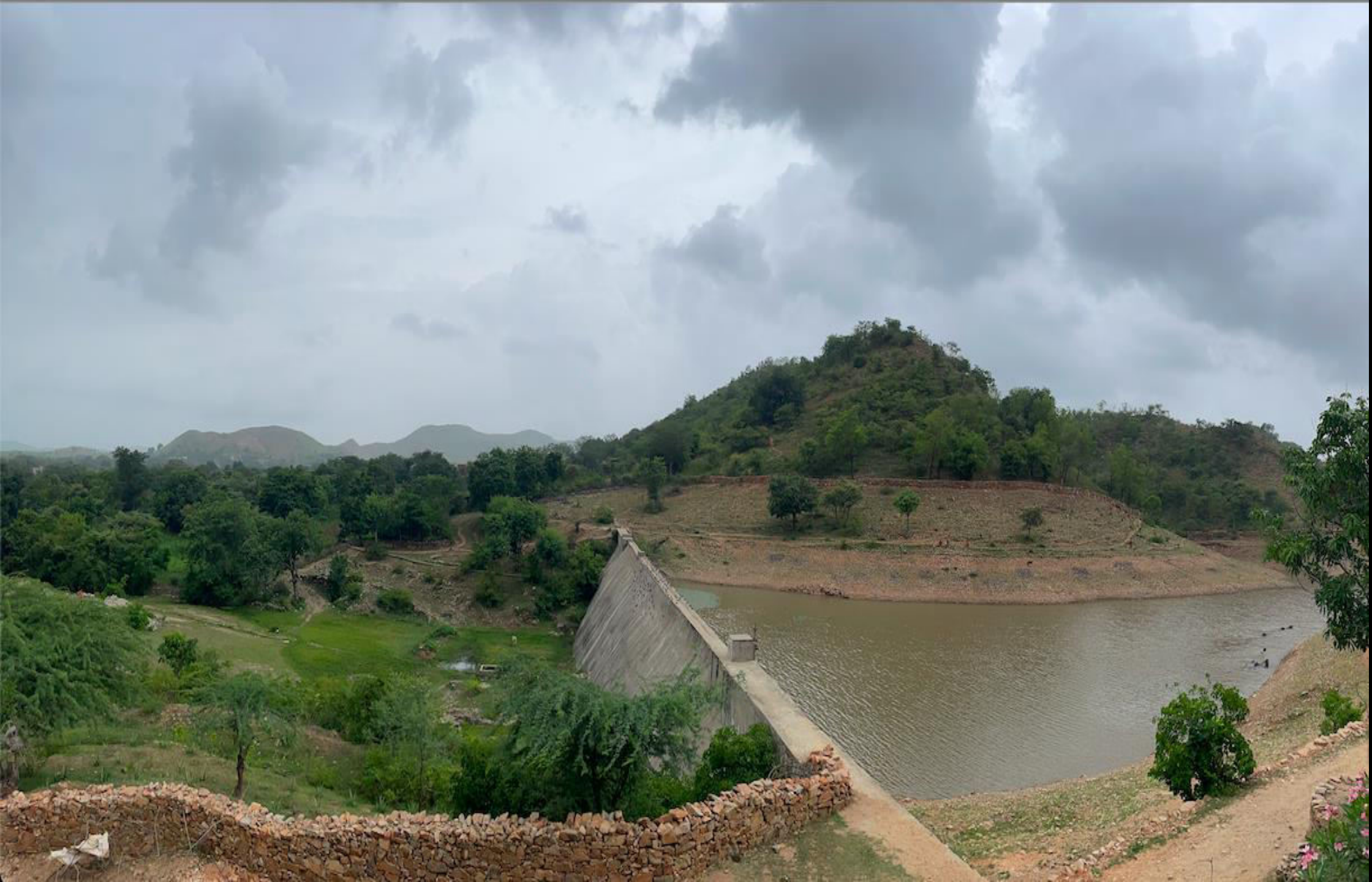
Image: Check dam and reservoir constructed under NREGA
