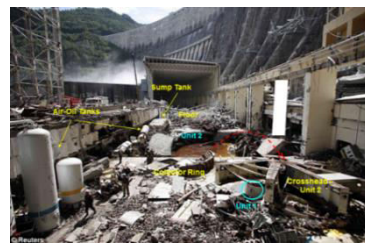
Safety management and risk control 安全风险管控
