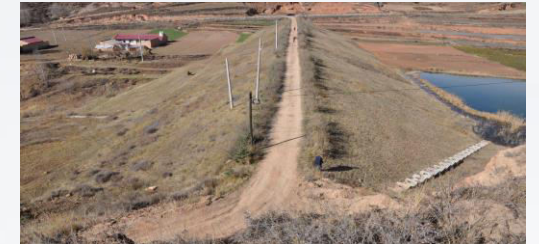
Silt arrest dam
