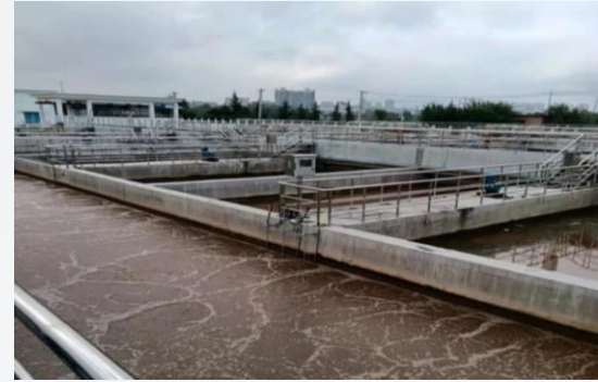
Centralized sewage treatment project
