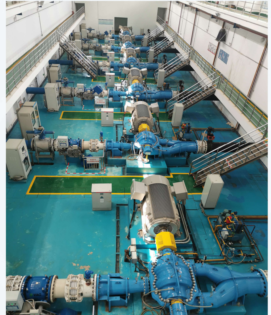
The horizontal middle-open multi-stage centrifugal pump group
