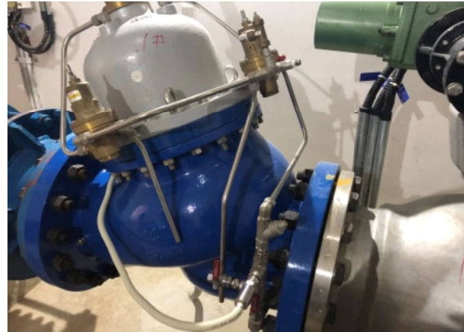
Water hammer prevention valve
