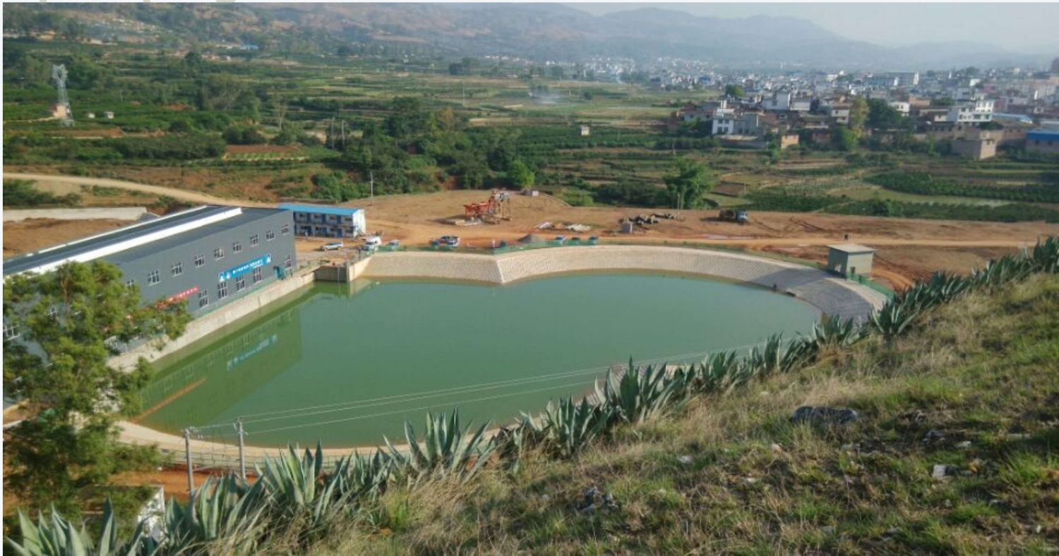
Panoramic view of primary pumping station
