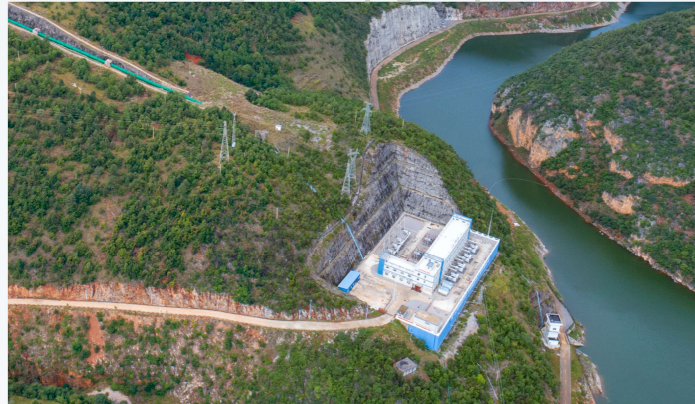
Project inlet—underground pumping station on cliff
