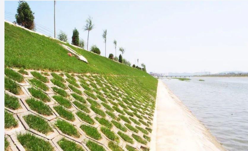
Ecological concrete revetment
