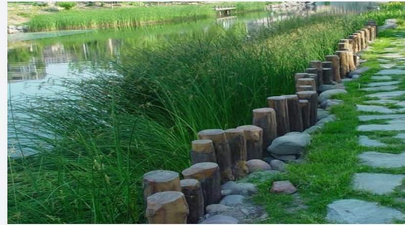
Wood pile or imitation wooden pile revetment
