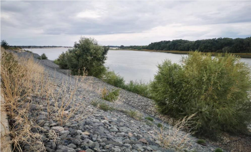
Stone gabion revetment
