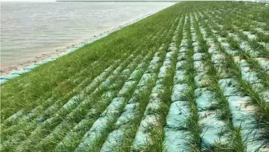
Ecological bag revetment
