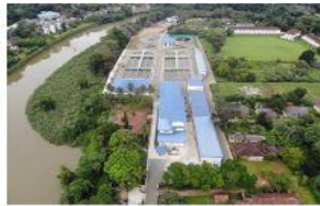
WWTP Oxidation ditch with capacity of 14,000m 3 /day
