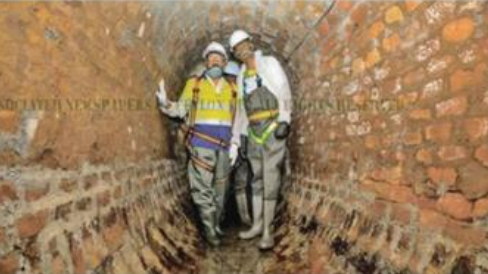
Minister Ranawaka inspecting the storm water tunnel.
