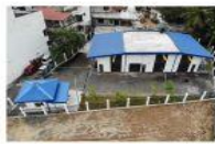
Main Pump Station (Package 01) At Heeressagala Junction
