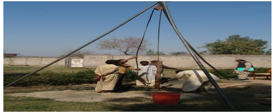
Installation of Exploratory Boreholes in the Field
