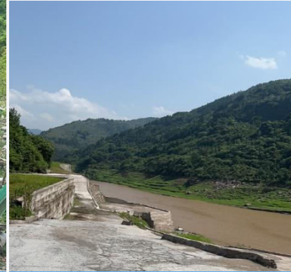
Abandoned dock in Pengxi River
