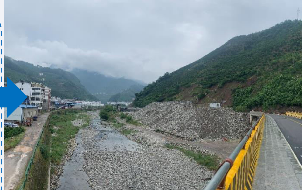
Quarry encroachment on river shoreline
