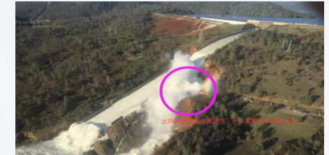
Spillway failure
