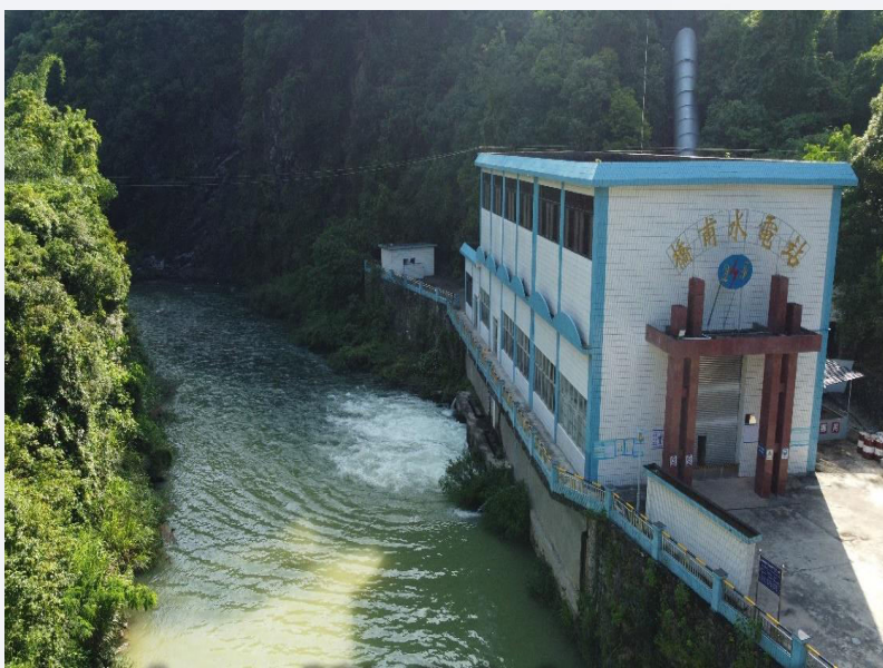
Powerhouse of QiaoFu hydropower station 桥甫水电站引水发电
