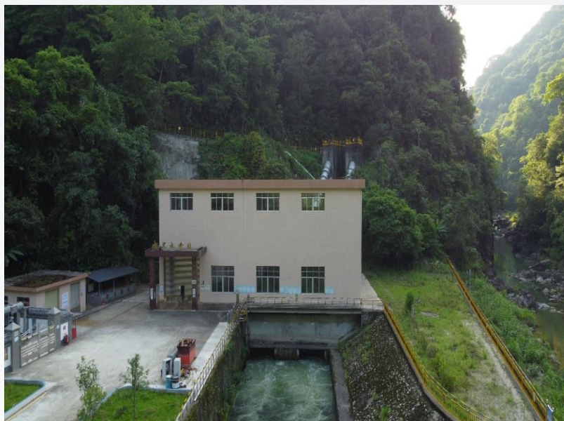
Powerhouse of BaMei hydropower station 坝美水电站引水发电
