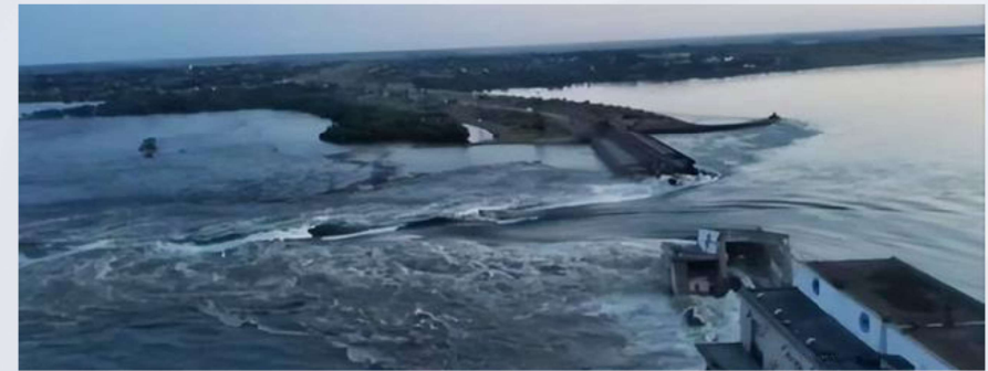
The breach of Kahovka dam
