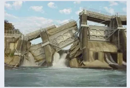
Dam break flood
