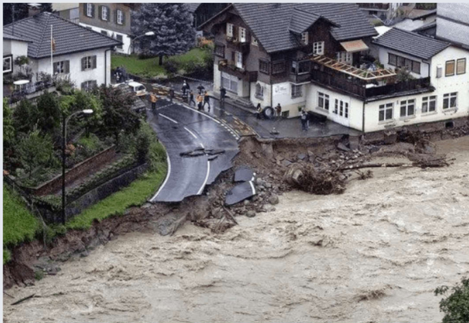
Flood destroyed buildings
