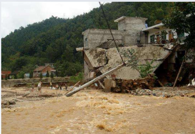
Flood destroyed buildings
