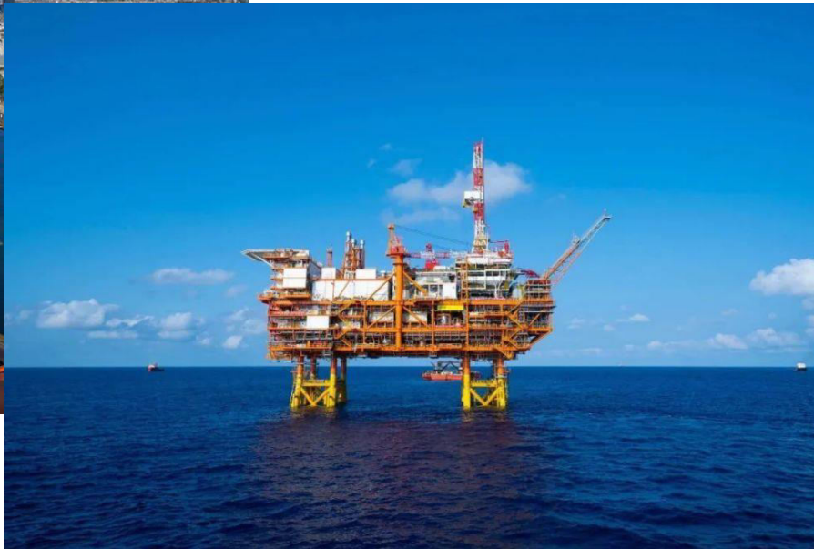
Oil platform (enping 15-2)
