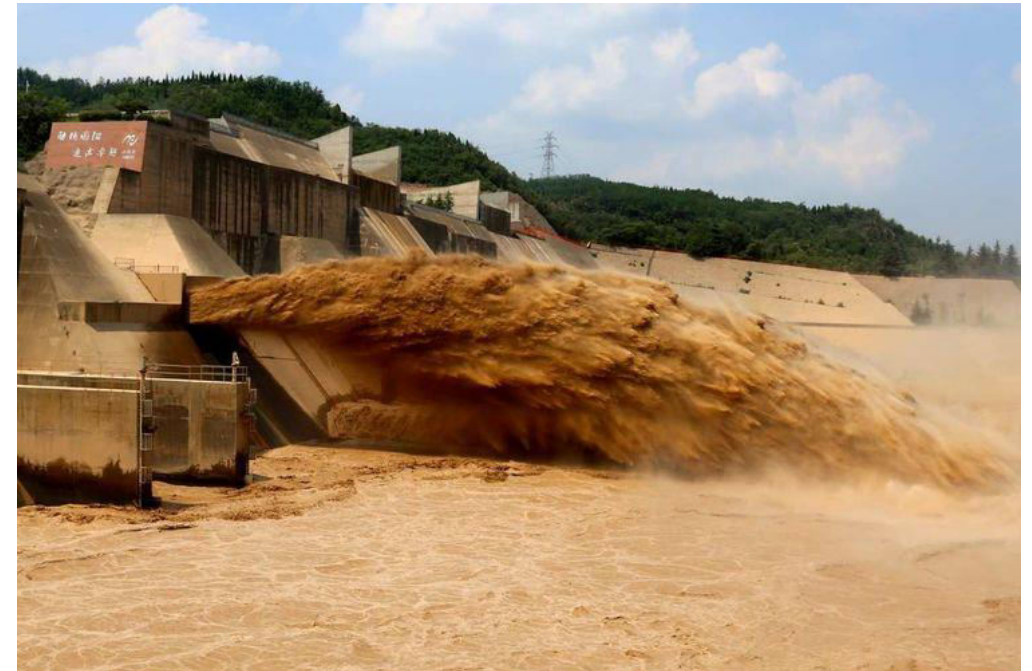
Sand removal of Xiaolangdi Reservoir
