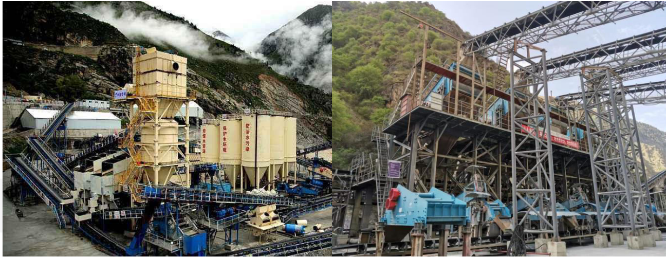
DG Aggregate Processing Plant Yebatan2#Aggregate Processing Plant
