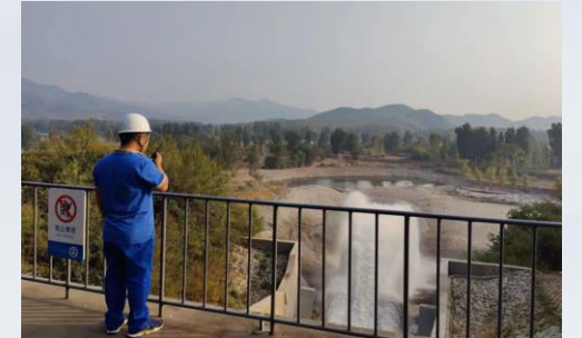
Water intaking from sandpits at Chaobai River
