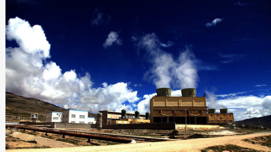
Geothermal power generation
