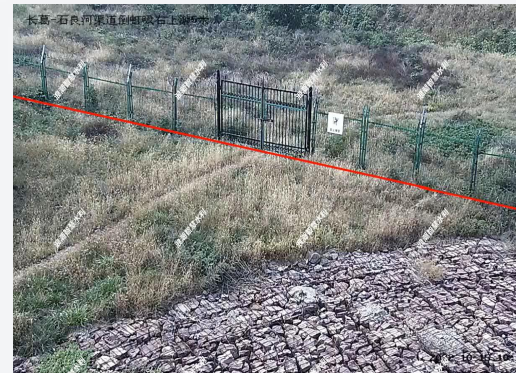
Trip line monitoring (fence perimeter)
