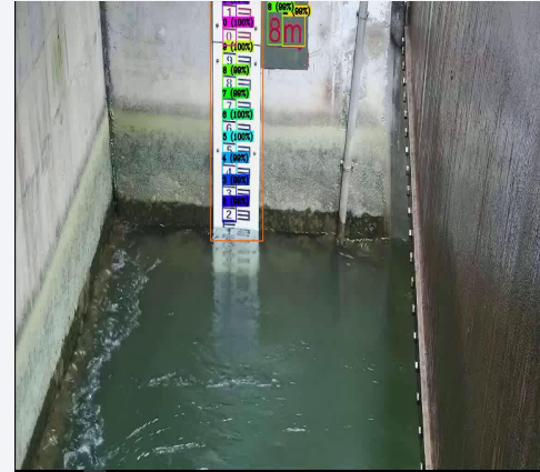
Water gauge reading
