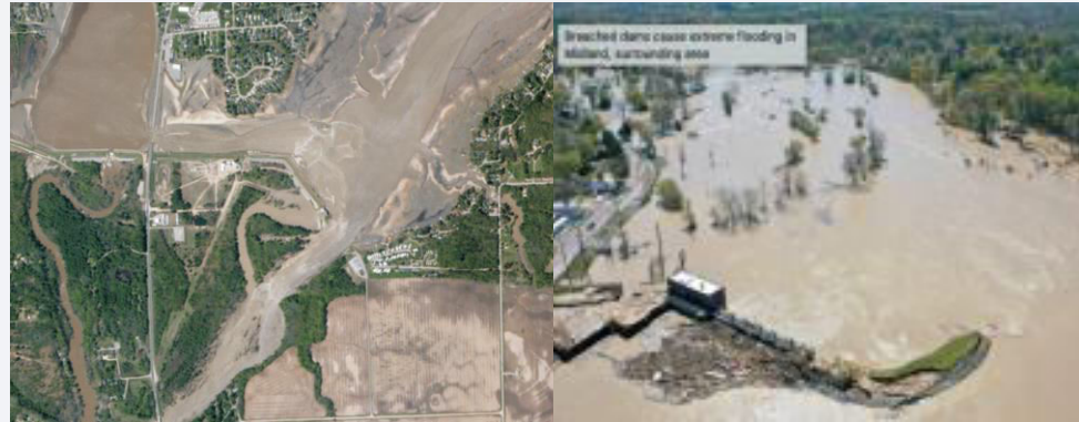
Sequential breaches of Edenville dam and Sanford dam (2020.5.19)
