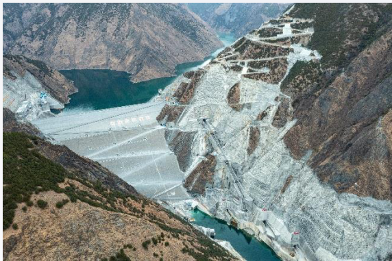
Lianghekou clay core rockfill dam
