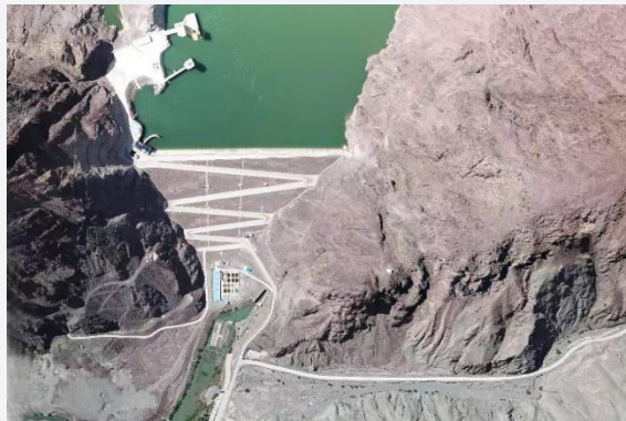
Chahanwusu concrete face rockfill dam
