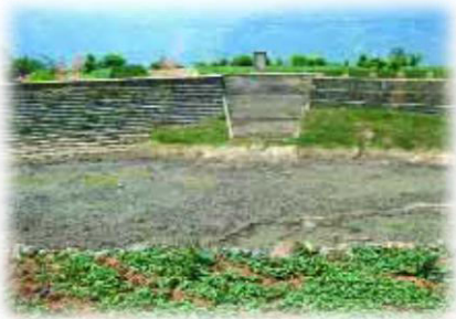
A dry water reservoir (Fengjie, Chongqing in 2006)
