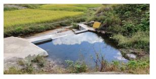
☐ Dug out:- Surface runoff water store and percolates in to the Ground.
