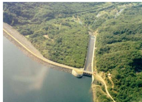
Image 7. Aerial view of the curtain and spillway
