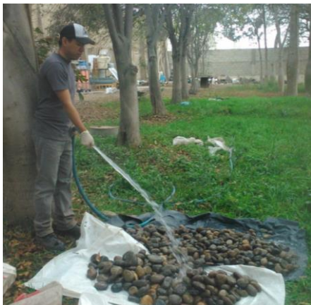
Figura 05.-Washing of gravel
