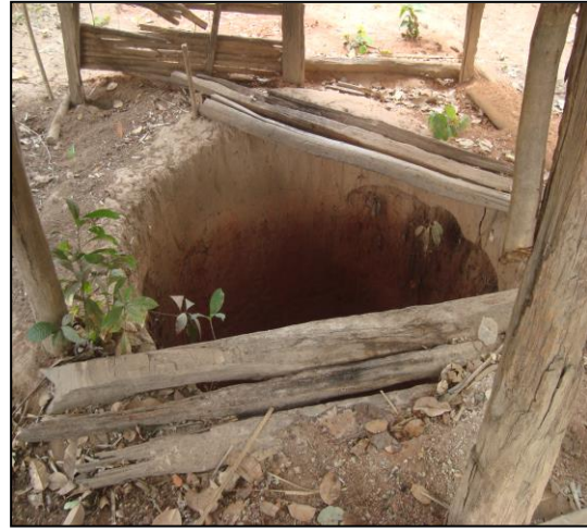
Figures 5 & 6 – Left: Simplified Water Distribution System; Right: A shallow open well dug by locals
