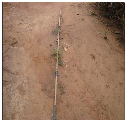
Figures 7 & 8 – Examples of pipes above ground and 'repaired' with rubber strips
