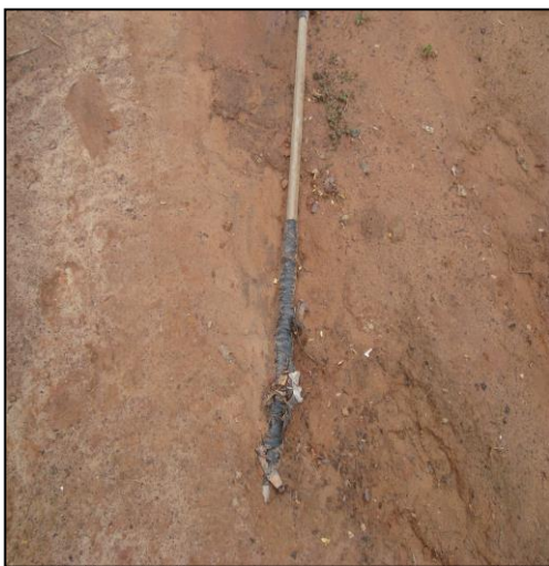
Figures 7 & 8 – Examples of pipes above ground and 'repaired' with rubber strips
