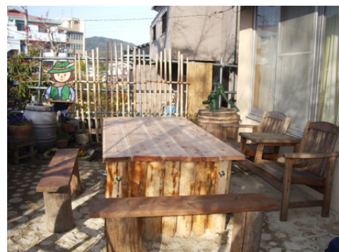
Fig.10 Installed a furniture type Rainwater tank
