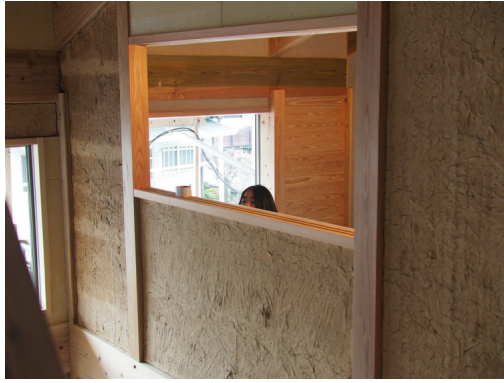
Fig.20 Making Earth Wall
