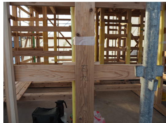
Fig.19 crosspieces and wedges through the Pillar
