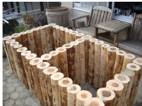
Fig.9 Building a Furniture type Rainwater Tank
