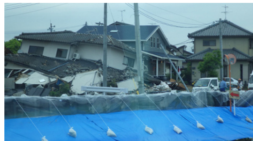
Fig.17 Damaged Buildings and Revee in Kumamoto Earthquake.
