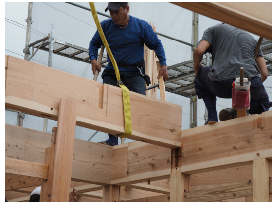
Fig.18 Beam and Pillar of SRH
