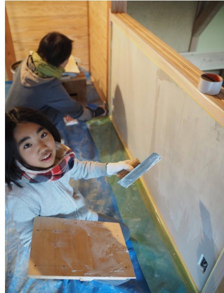
Fig.21 Plaster on Earth Wall
