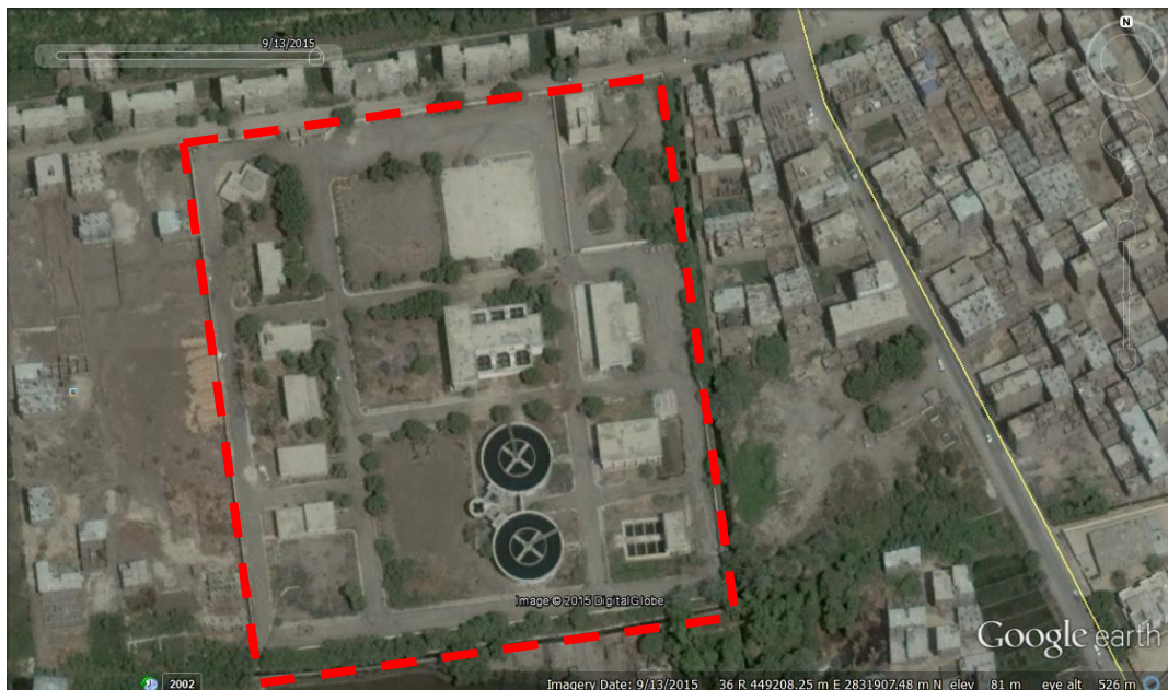
Figure 1.0 Satellite image for Armant WTP (34,000m 3 /day), Qena, Egypt.
