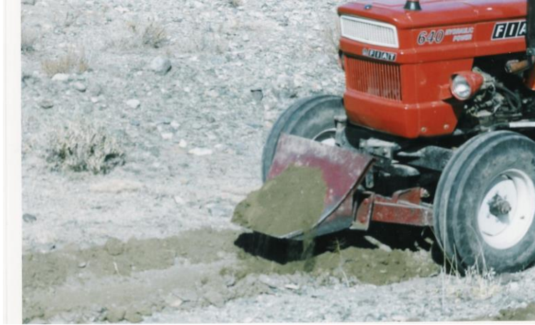
Figure 6: Pit Maker for making pits in ditches
