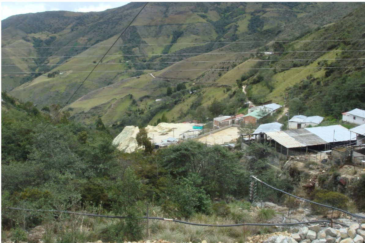
Figure 2 General view of the "Reina de Oro" gold ore beneficiation plant, located in Vetás Municipality, Santander, Colombia
