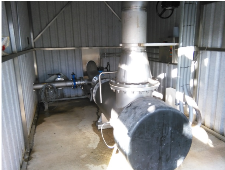
Figure 4: Tertiary process water treatment system on-site at the Kerry Group dairy plant, Listowel, Co. Kerry
