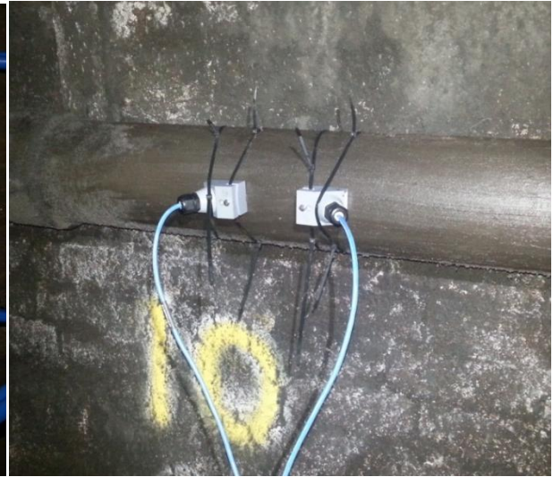
Figure 8: The transducers clamped onto the discharge pipe
