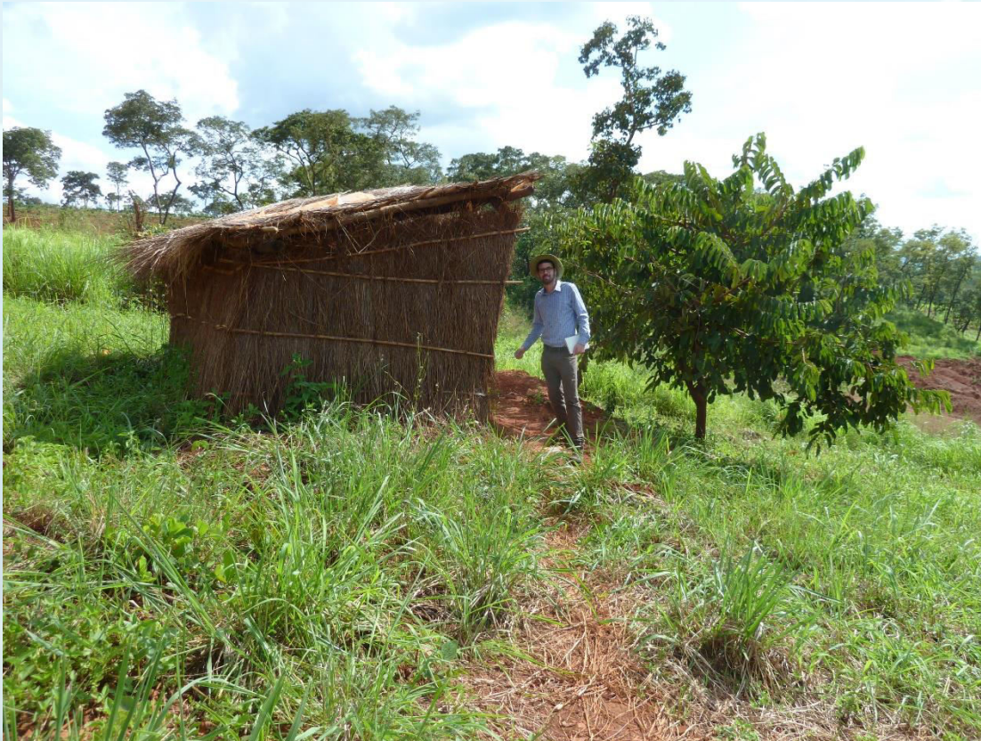
Inadequate WASH provision
